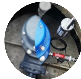
AQS-Edge Hydrophone for Below Ground Installation
